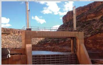
This spillway is operated by two  $\emptyset 8" \times 120"$  stroke, flange-mounted, mill-type actuators with a  $\emptyset 4"$  high-strength, stainless steel piston rod, and protected from the outdoor elements by special paint.
