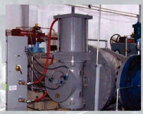
Ø18.00" actuator has a Ø4" stainless steel piston rod with a 4" stroke adjustment rod operates a Ø30" cone valve via a light hydraulic control panel.
